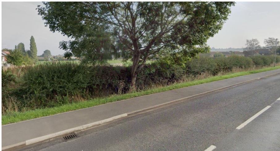
Photo 3: Pedestrian Infrastructure on Station Road
