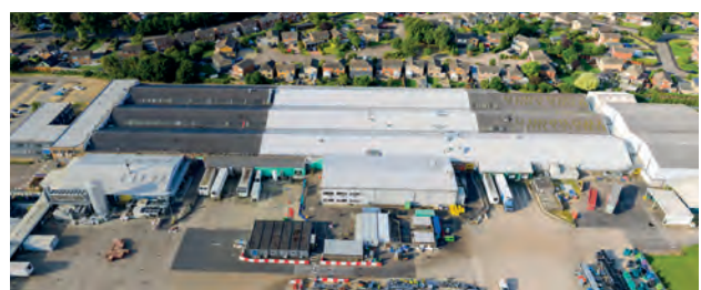
New over-roof in situ
